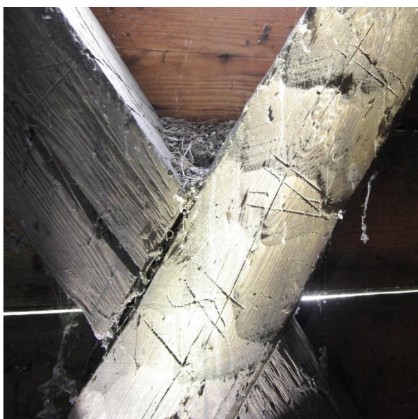
Fig.6 Marks in a church in Grodziec on the top truss beam of the construction.
