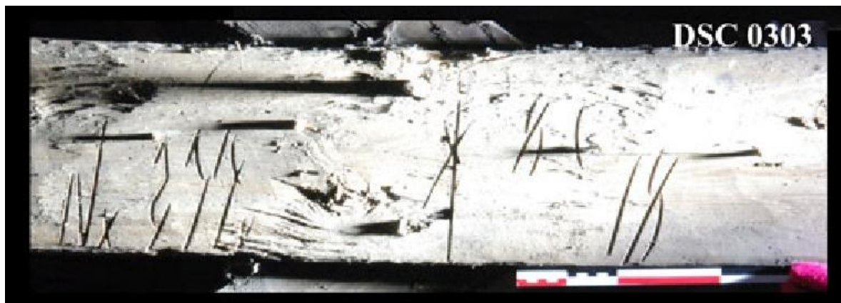
Fig . 9 Commercial sign on the roof frame of middle 19th c tenant house in Brussels (photo: ©MRBC-DMS; CEA/ULg; KIK-IRPA).
