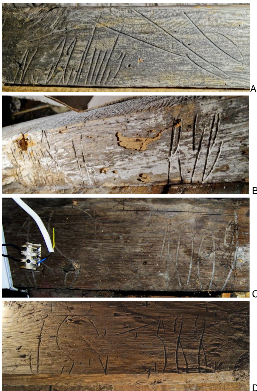
Fig. 8 Signs on the rafters of tenant houses at 21a,C,D 3 rd of May Street in Gdansk (photo M. Jedlikowska)
