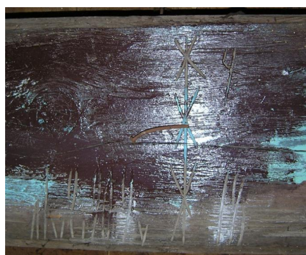
Fig.7 Signs on the rafters in tenant houses at 3 rd of May Street in Gdansk - photo M. Jedlikowska
